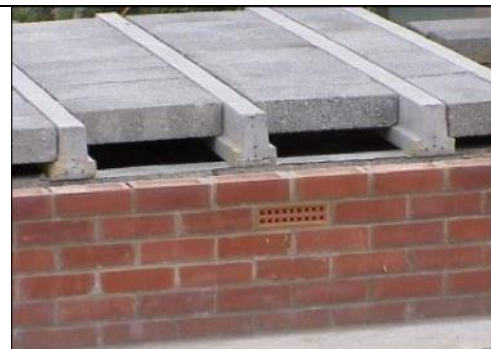
Figure 1.4 A beam-and-block ground floor. The wall below the DPC, often includes an airbrick. This ventilates the empty space below the suspended floor.
